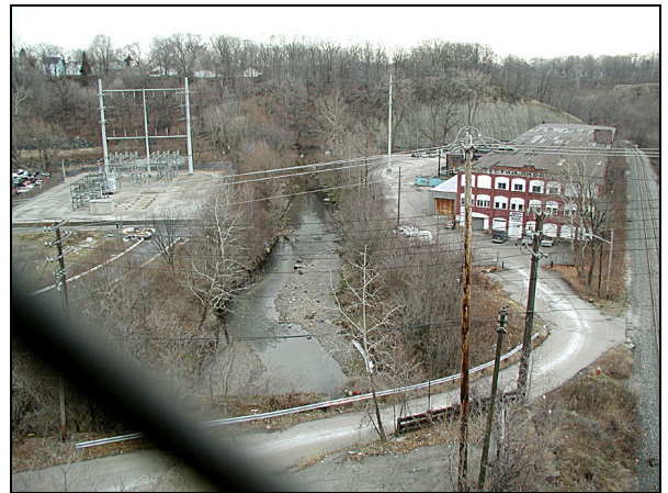
Industrial Facility below US-42
