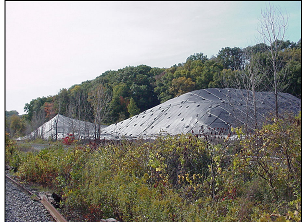
Road Salt Storage Site lies to north of Stream
