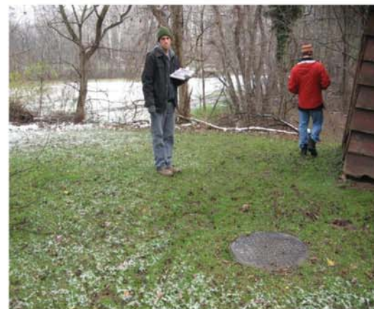
Manhole leading to the underground pipe that will be diverted to treatment areas.
