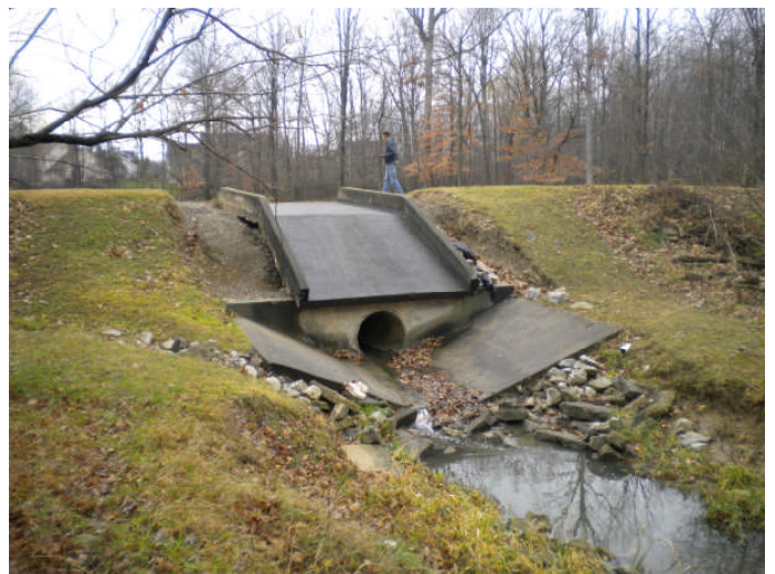
View of outlet structure at north end of basin
