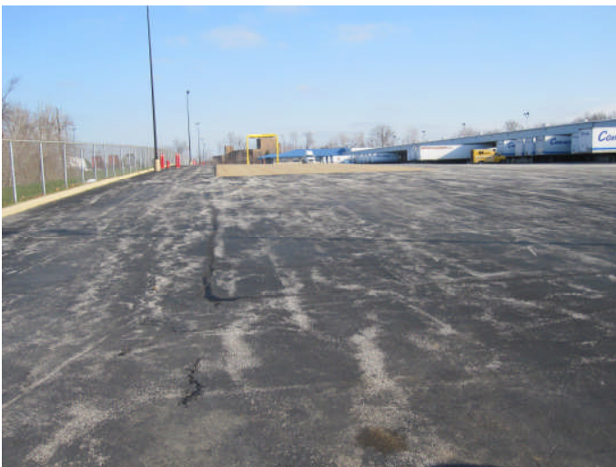
View of parking lot from northwest corner
