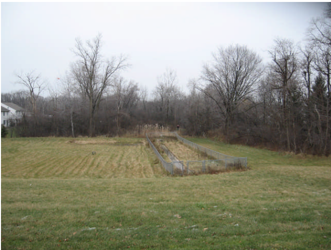
View of swale from parking lot
