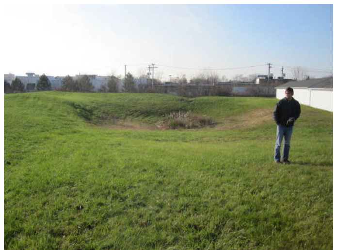
View of basin from Giant Eagle
