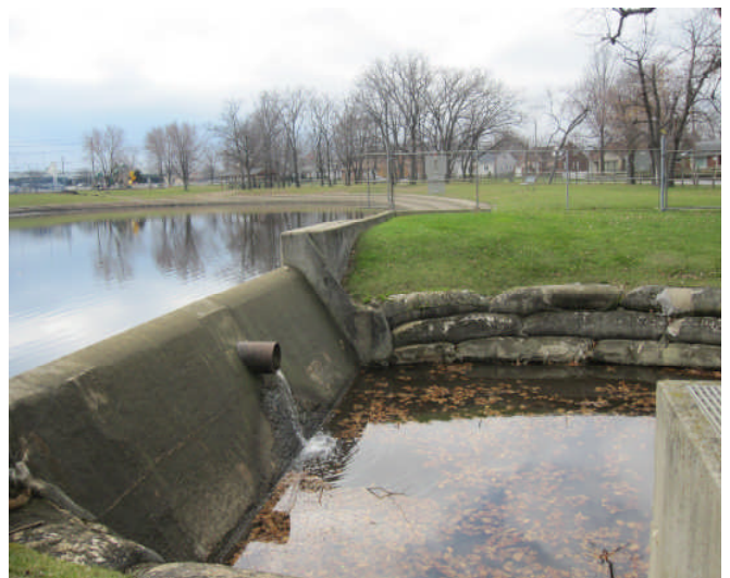
View of outlet structure from northwest end
