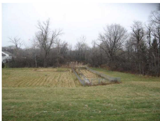
View of swale from parking lot
