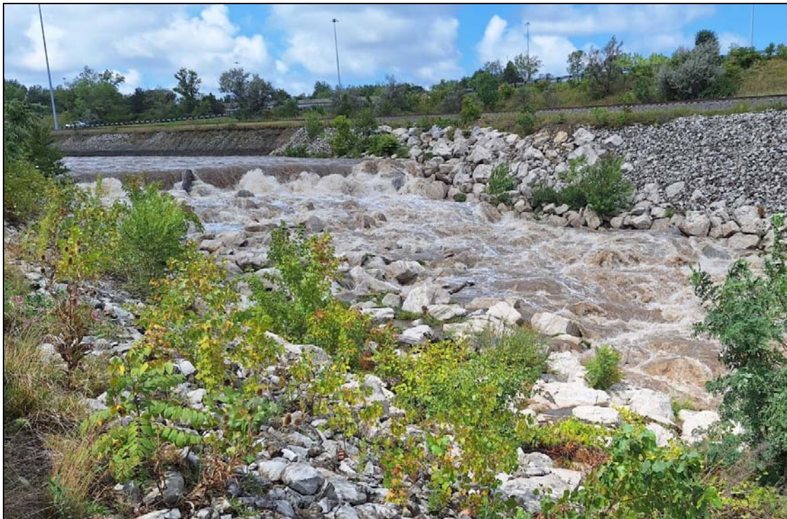
Big Creek Spillway, Brookside Reservation, August 2024, after 2019 modification
