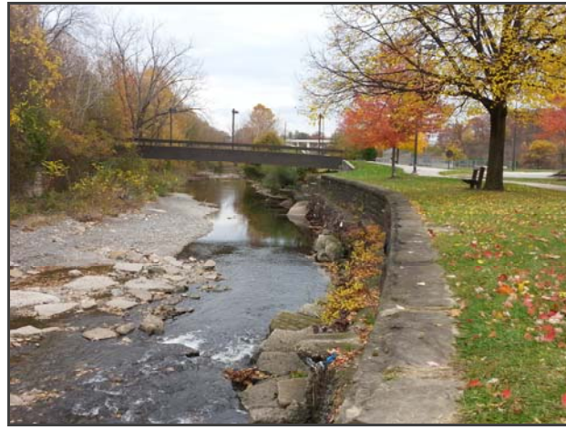
Brookside looking east from drop structure area with proposed trail alignment to the right
