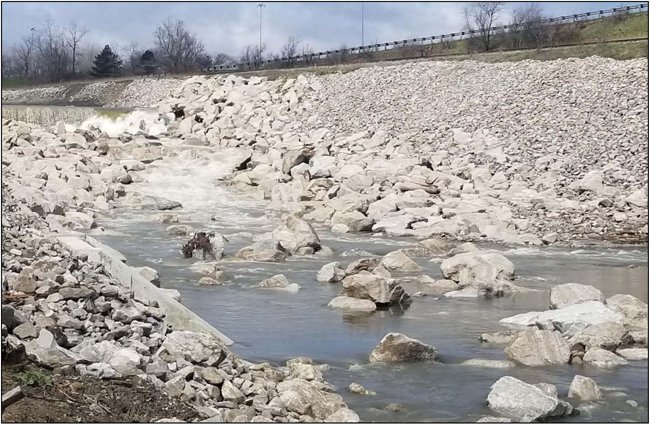
Figure 33: Brookside Spillway photo – Existing
