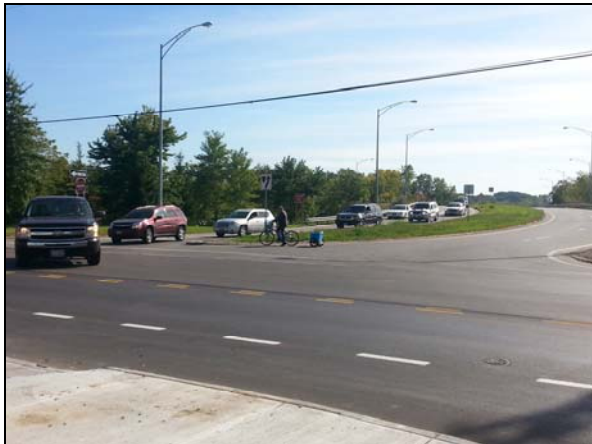
Denison Avenue Access ramps looking south
