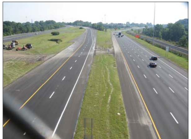
I-71 looking east from Ridge Road bridge
