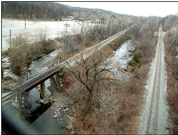
Norfolk Southern and CSX Railroads Rights of Way Parallel the Creek
