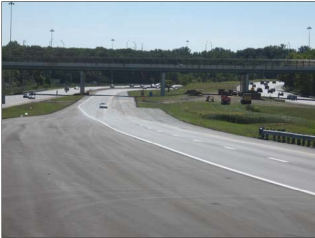
I-71 / Denison Exit Ramp looking west towards Ridge Road bridge
