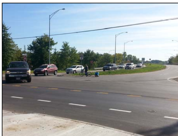
Denison Avenue Access ramps looking south
