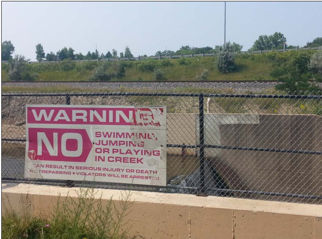
Big Creek Drop Structure, Brookside Reservation
