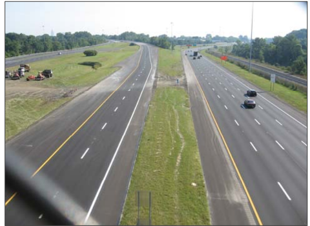
I-71 looking east from Ridge Road bridge
